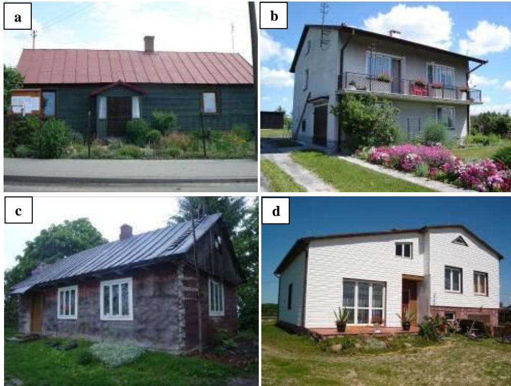
Photo 3. Wall cladding in houses: a-coating, b-plasterwork, c-tar paper, d-siding (Source: author's photographs).
