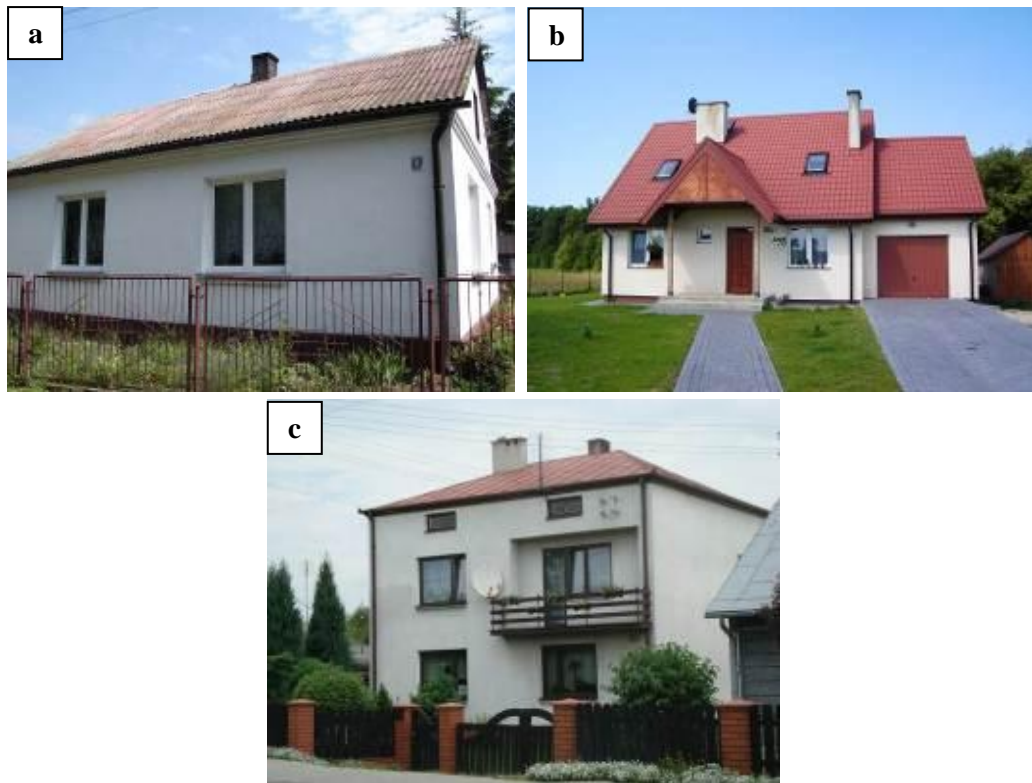
Photo 4. Examples of houses: a-one-storey, b-with functional loft, c-two-storey (Source: author's photographs).
